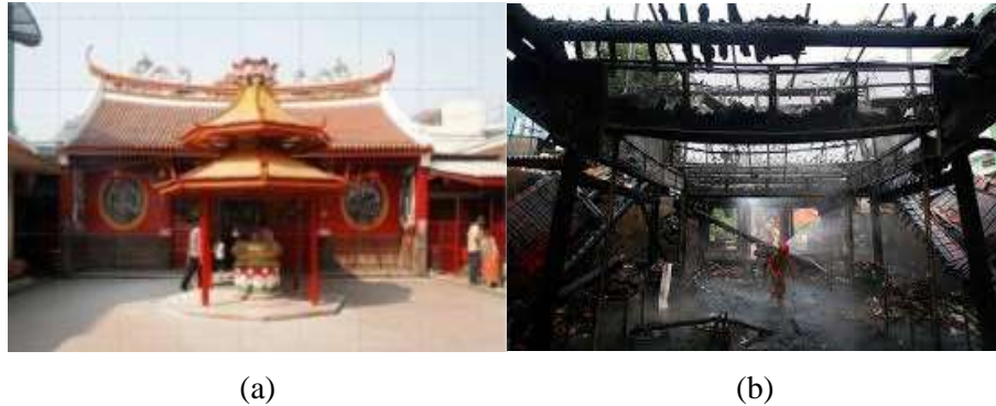
Figure 1 Condition of Dharma Bhakti Monastery: (a) before and (b) after burning. (source: Management of Dharma Bhakti Monastery)
