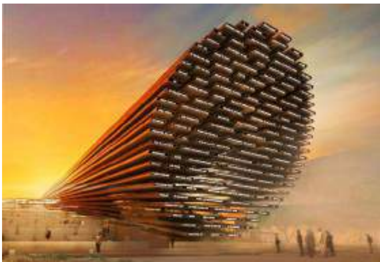
UK Pavilion-Expo 2020 Dubai
