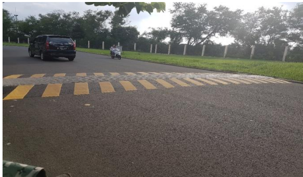
Figure 7 Observed Segment with Standard Road Hump
