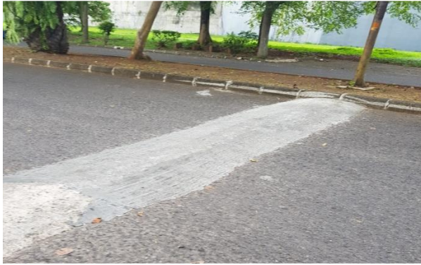
Figure 8 Observed Segment with Non-Standard Road Hump
