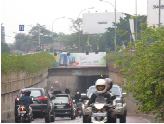
Figure 2 View of the Underpass Taken from Simprug
