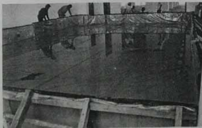
Gambar 14. Proses pengisian beban air
