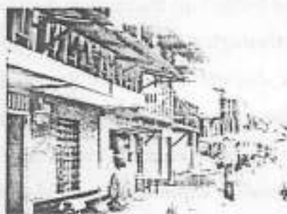
b. Row of renovated houses
