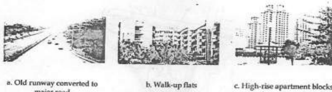
Figure 5-2 New facilities in Kemayoran New Town
