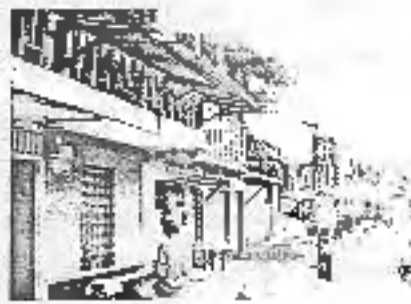
b. Row of renovated houses
