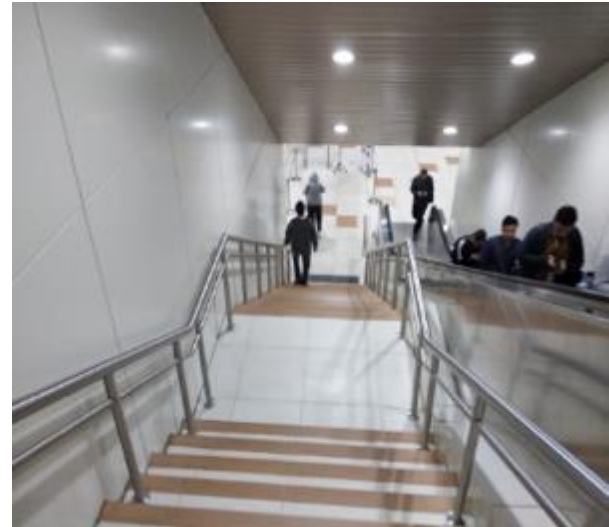
Figure 3. The Section of Stair from the Concourse Floor (B.1) to the Platform Floor (B.3) Source: Authors, 2019
