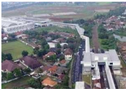
Figure 8 Skybridge. Source: StasiunCisaukjadipeluangemaspengembang, Dwytia Putra, 2019
