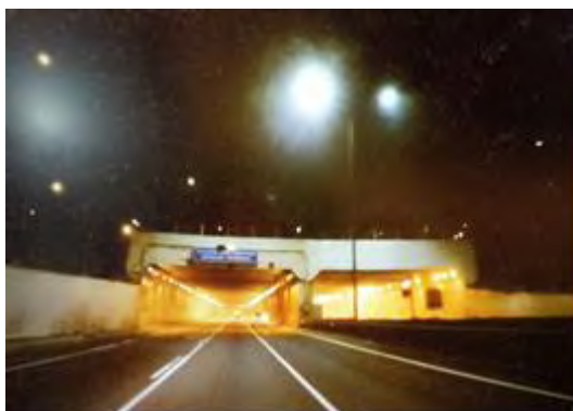
Fig.1 Pasar Rebo tunnel at night [4]
