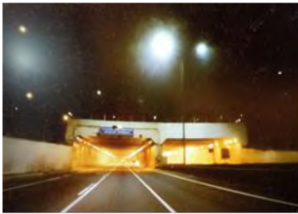
Fig.1 Pasar Rebo tunnel at night [4]
