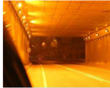
Fig.2 Wall mounting asymmetrical lighting [4]
