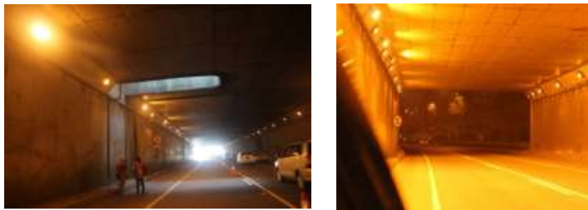
Figure 3 Pasar Rebo Tunnel with flat ceiling shape
