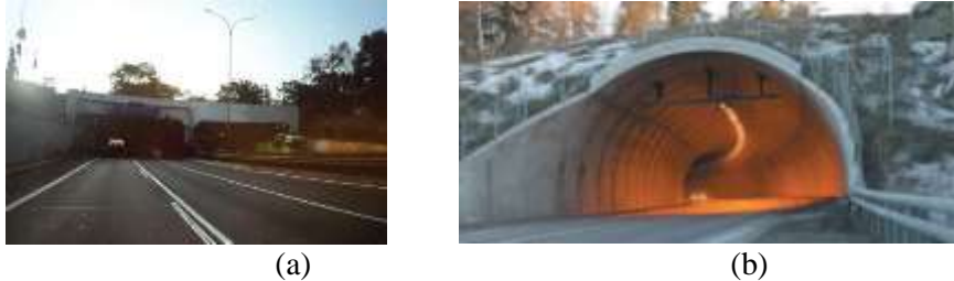
Figure 2 (a) Access Zone of Flat Tunnel – Pasar Rebo Tunnel [6] (b) Access Zone of Arched Tunnel [7]
