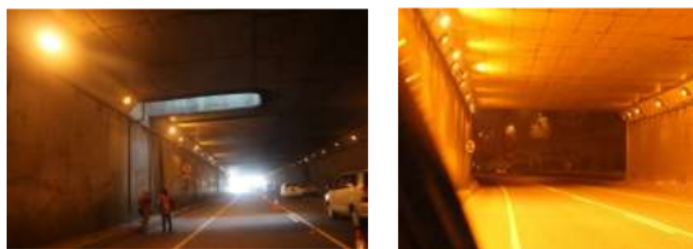
Figure 3 Pasar Rebo Tunnel with flat ceiling shape
