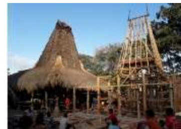
c. House Construction Process (August 2019)
