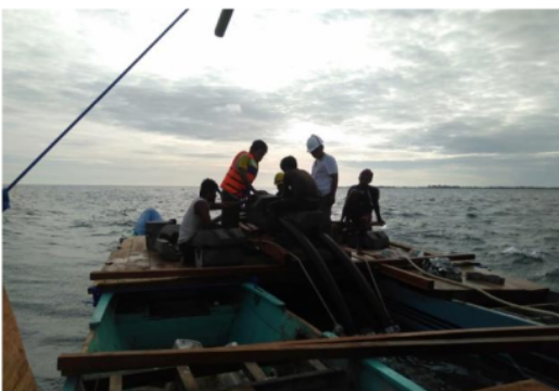
Figure 12. Underwater pipe installation process with TJ-19 method
