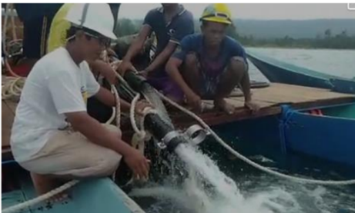
Figure 9. Drain pipe before connecting
