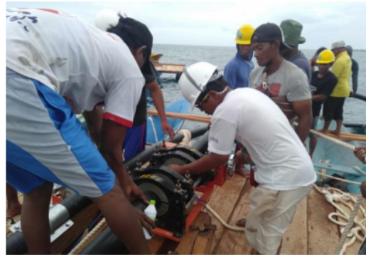
Figure 10. The process of connecting pipes on ships/boats
