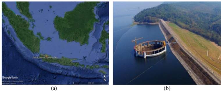
Fig.1. (a) Location of Jatiluhur Dam in Java Island, Indonesia. (b) The Rock-fill Jatiluhur Dam (photo: perusahaan jasa tirta II.)
