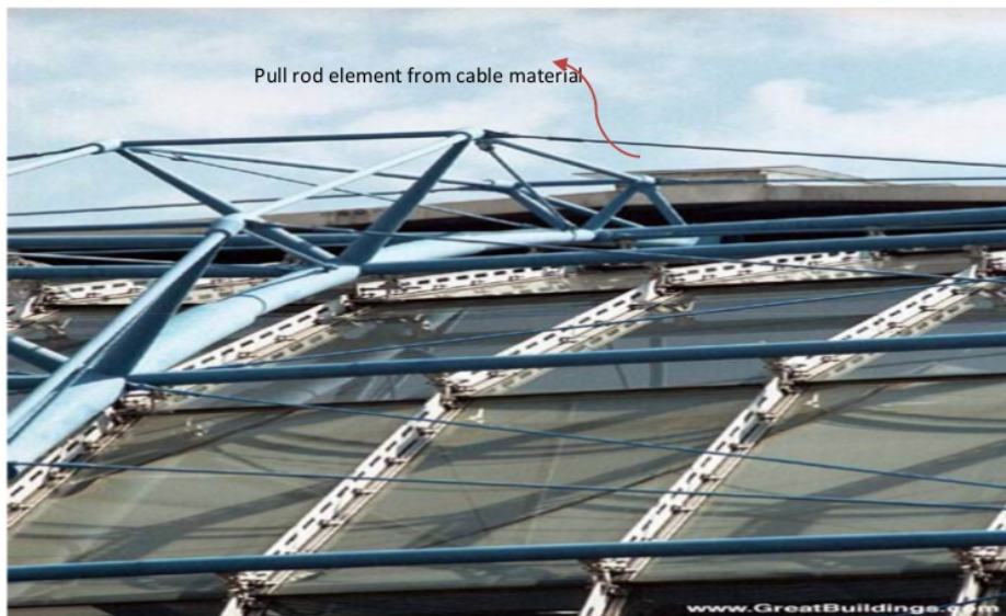
Figure 5 The Use of Cable Material for Pulling Rod in Truss Structure
