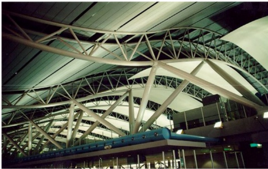
Figure 9 The Example of Truss Space Structure System, Kansai Airport, Osaka, Japan.
