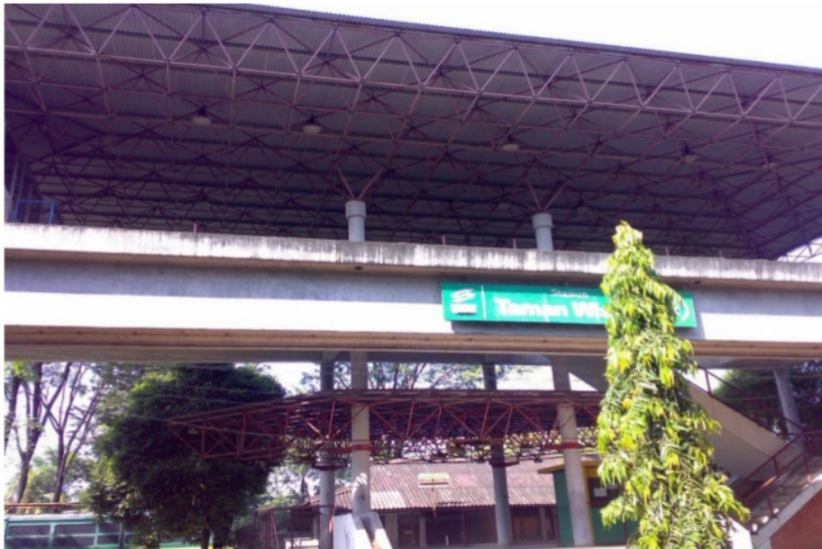
Figure 10 the Example of Space Frame Structure on the Roof of a Building in Taman Mini Indonesia Indah, Indonesia
